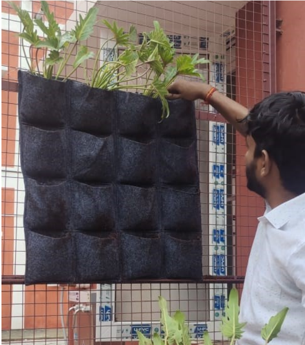
Fig. 1. Setting up a felt - integrated living wall.
