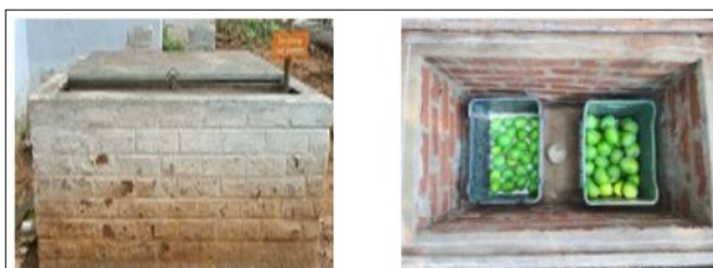
B. Zero energy cool chamber.
