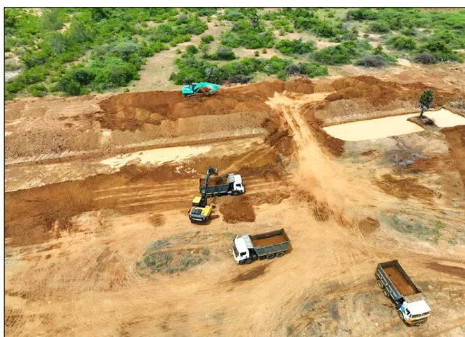
Fig. 5. Desilting work at Udaikulam Kanmai led by Siruthuli NGO to enhance water storage and drought resilience (54, 55).
